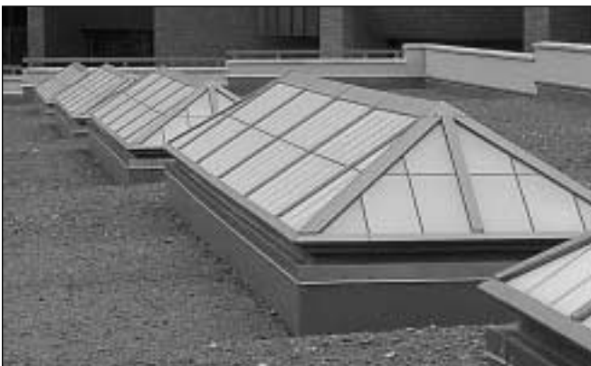
Skylights allow diffused light into Cofrin Hall classrooms
