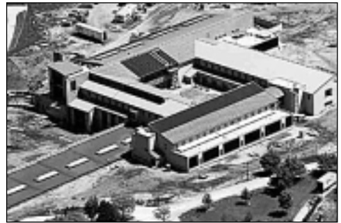
Cofrin Hall under construction
