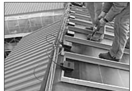
Standing Seam Metal Roofing being installed
