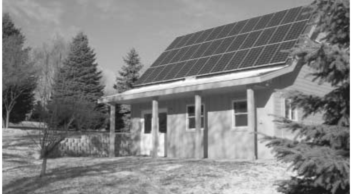
A garden shed doubling as a solar power plant. The 36 solar electric panels on the roof provide enough power to run all the appliances in the Wilcox home—including air conditioning. Surplus electricity is sold back to the local utility.
