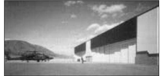
Preheat Solar Collectors on a Plane Hangar
