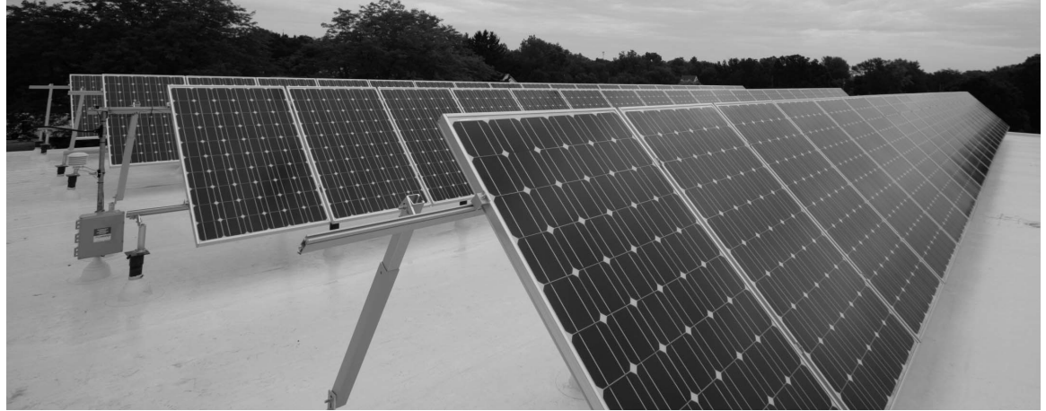
One of many projects led by Dennis Kuchenmeister, director of buildings and grounds, this 19-kilowatt solar electric system was installed at Purdy Elementary School.
