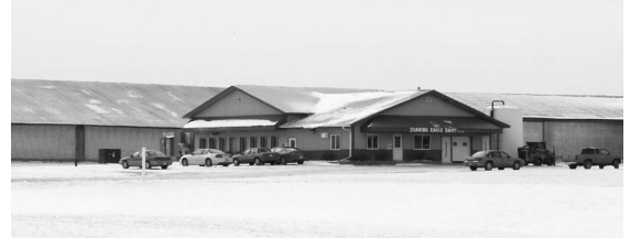
Soaring Eagle Dairy animal housing and milking facilities.
