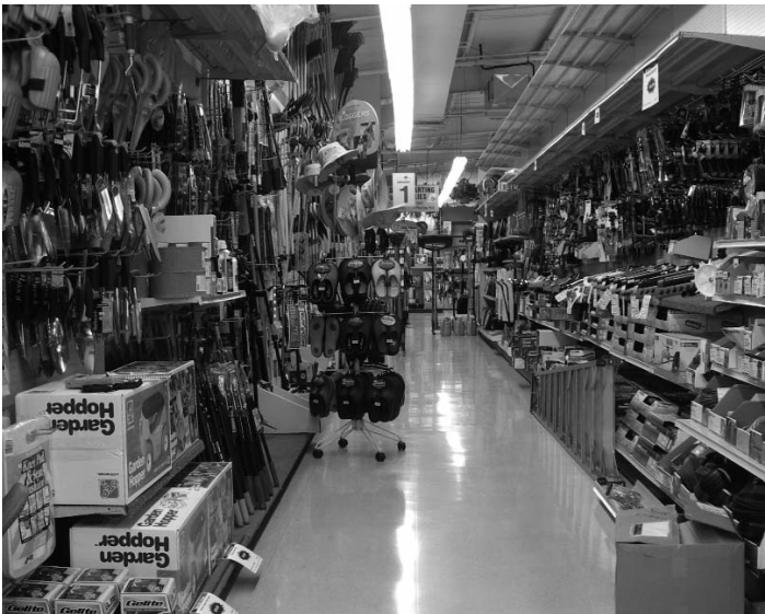
Store aisle after lighting upgrade
