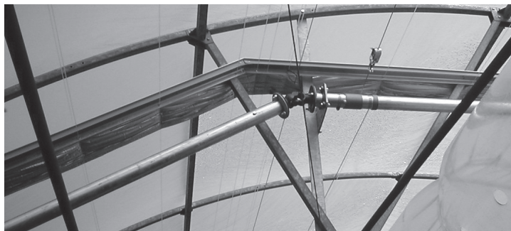
The mechanical system of the energy curtain makes deploying and retracting it an easy process. The energy curtain is automatically controlled and uses a small electric motor to open and close the curtain.
