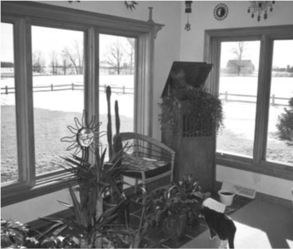
Double-pane low-e windows reduce both infiltration and heat loss while admitting both light and heat from the sun. Ceramic floor tile provides some of the home's thermal mass by absorbing and radiating solar heat.
