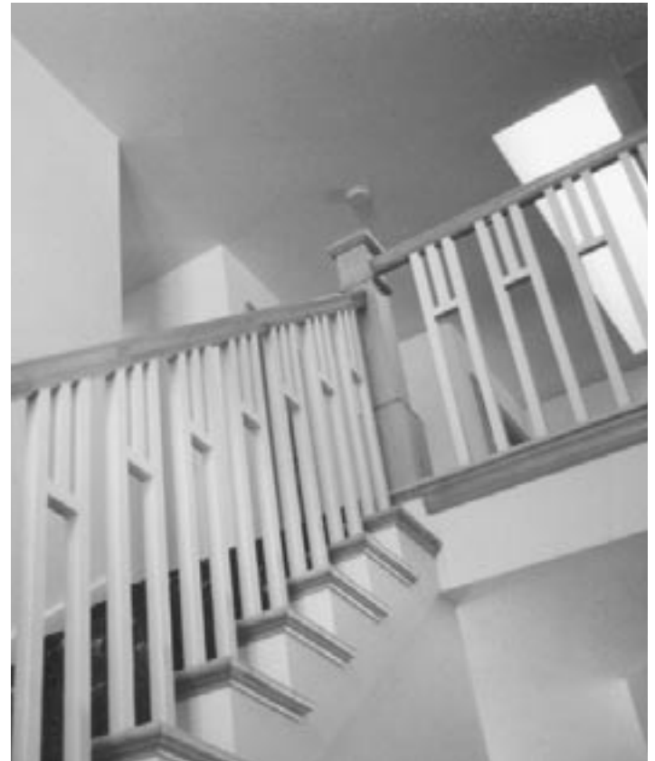
This skylight in the upstairs hall augments the home's daylighting strategy and draws visual attention to the elegant staircase.
