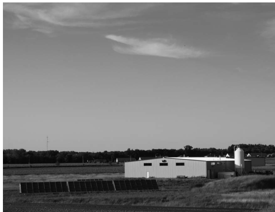
Central Waters Brewing Company in Amherst, Wisconsin installed a 24 panel solar hot water system in March 2009.
