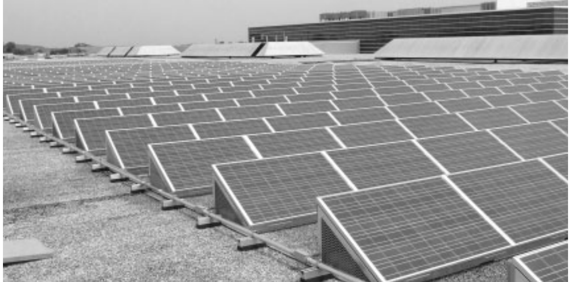
Photo 1: The 135kW solar electric system mounted on the flat roof of the GE Health Care building in Waukesha, Wisconsin, is held in place by ballasted racks. No penetration of the roof membrane was needed.
