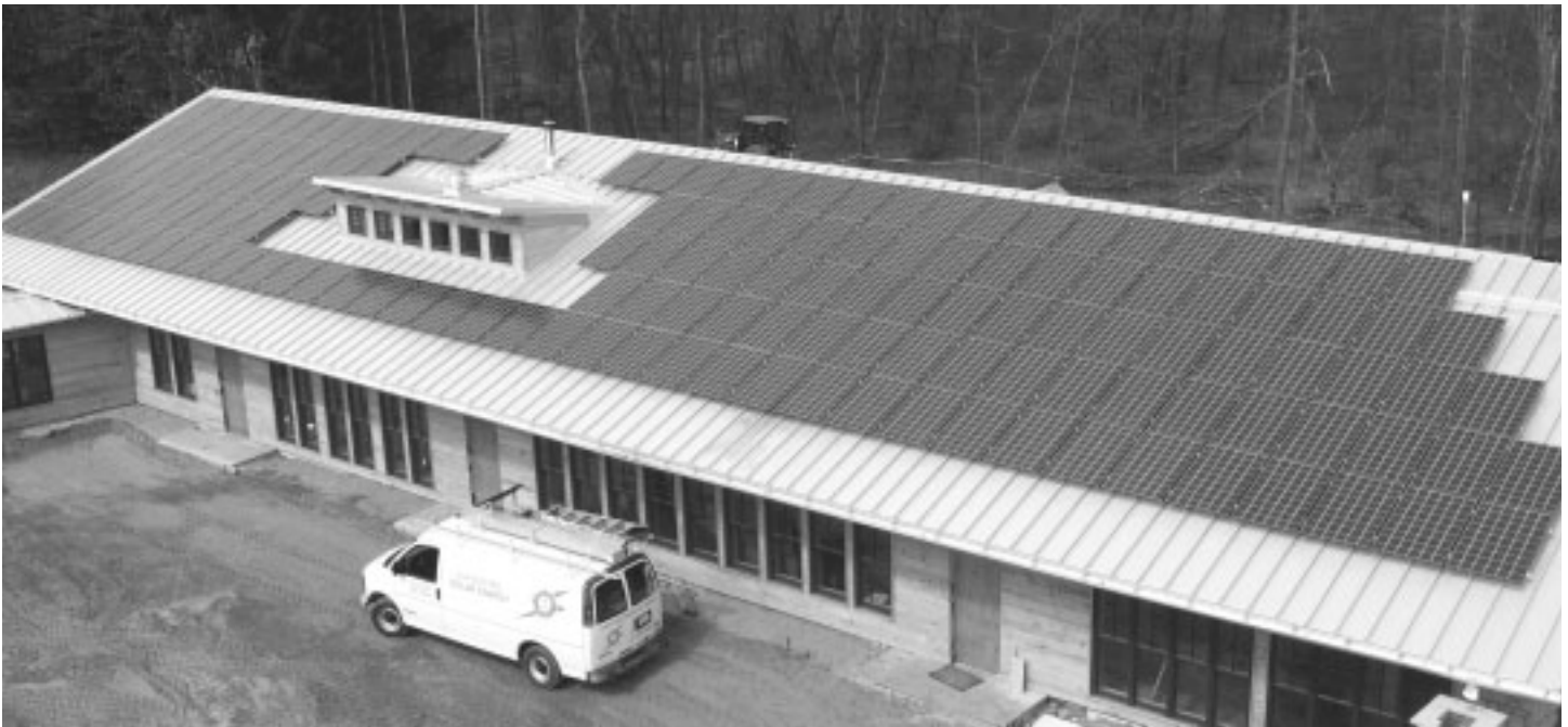
Photo 2: The Aldo Leopold Center in Reedsburg, Wisconsin, expects to get 110 percent of its electricity from the 39.6kW solar electric system that is flush mounted on its sloping roof. Connected to the electric grid, the system will produce extra electricity in the summer which can then be drawn back from the grid during the darker winter months.
