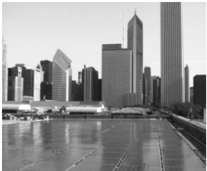
Photo 5: This 130kW solar electric tile system is located atop the Art Institute of Chicago.
