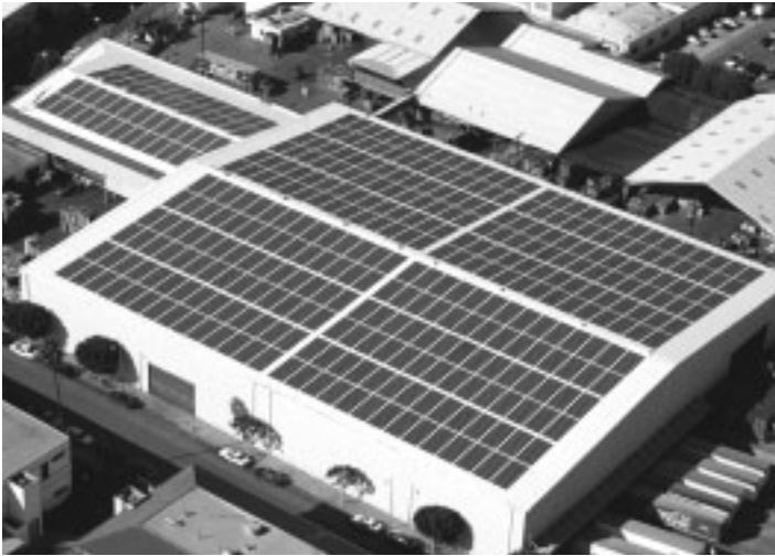
Photo 4: Thin film solar electric modules installed directly to the surface of this roof provide 325 kilowatts of electricity for the Coca Cola bottling plant in Los Angeles, California.
