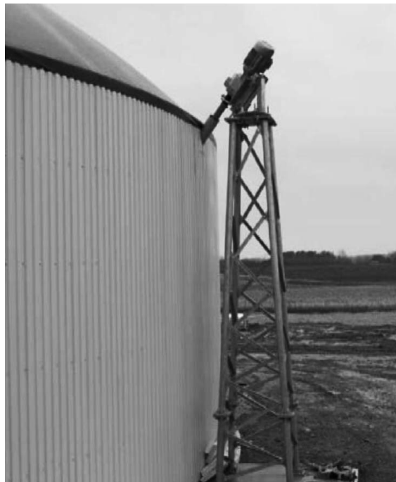
Clear Horizons' patented mixing technology combines cow manure with waste cheese whey from the Crave Brothers dairy and cheese operations to produce significantly more biogas than a manure-only digester.
