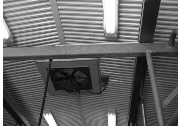
With the assistance of Focus on Energy, the farm installed energy-efficient lighting that will save the farm almost 24,000 kilowatt hours annually.
