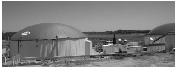
Crave Brothers Dairy Farm added a second digester tank to keep up with the farm's growth.
