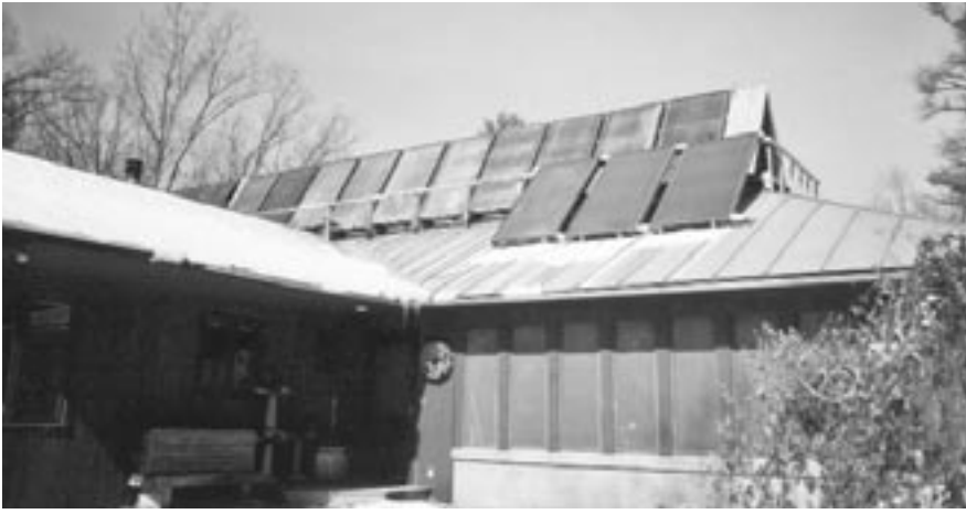
(above left) Thirteen solar thermal panels heat water for space heating and domestic use. The photovoltaic panels that generate one-third of the Davenport's electricity are located at the west end of the roof (out of view). (above right) All windows in the Davenport home are triple glazed low-e units except those on the south side, which are low-e double-glazed to admit more sun.
