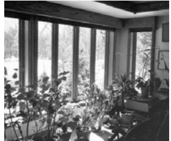
(above left) Thirteen solar thermal panels heat water for space heating and domestic use. The photovoltaic panels that generate one-third of the Davenport's electricity are located at the west end of the roof (out of view). (above right) All windows in the Davenport home are triple glazed low-e units except those on the south side, which are low-e double-glazed to admit more sun.
