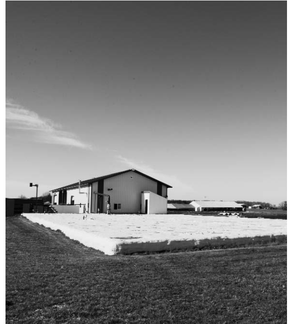
Quantum Dairy near Weyauwega, Wisconsin, employs a modified plug-flow digester system to produce enough energy to power 325 average Wisconsin homes.
