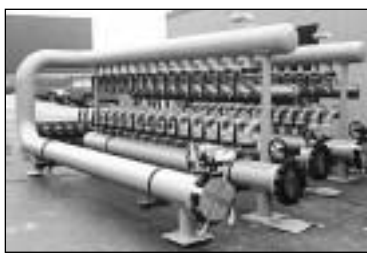
Photo above: Header valve assembly to be placed in valve pit.
