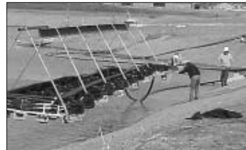
Coil assembly raft being placed in one of two man-made ponds.
