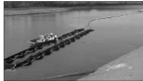
Photo above: Preparing to sink the loop assembly raft.
