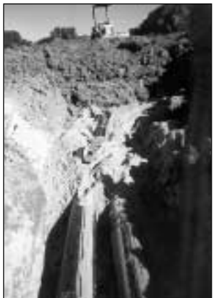
10-inch supply and return lines were laid.
