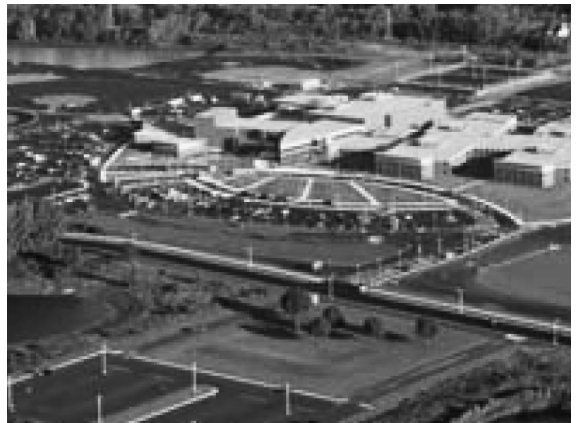
This high school in Fond du Lac, Wisconsin uses a ground source heat pump system (pond loop) for heating and cooling.
