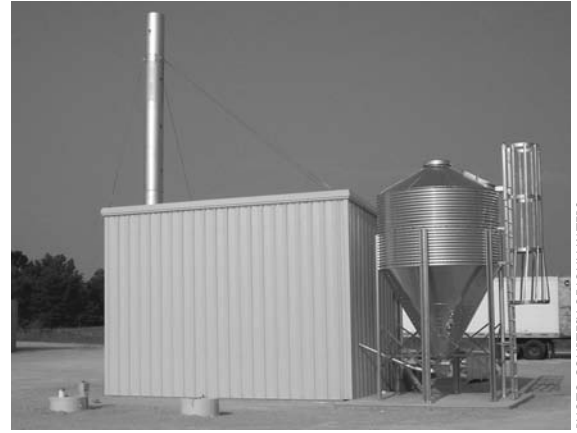
Underground pipes connect the biomass boiler to the building heating system. The hopper that feeds the wood fuel to the burner is shown on the right.
