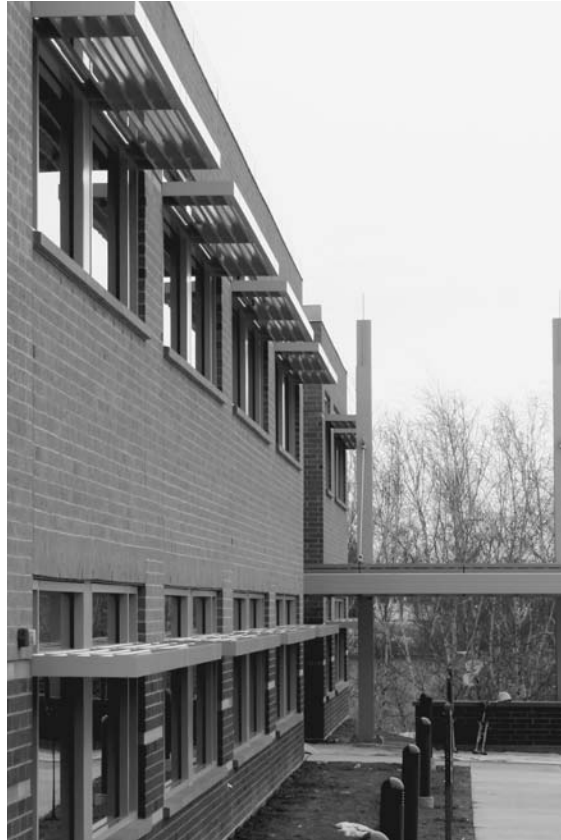
Daylighting louvered sunscreens direct light far into the interior office spaces at the Wisconsin Energy Conservation Corporation.
