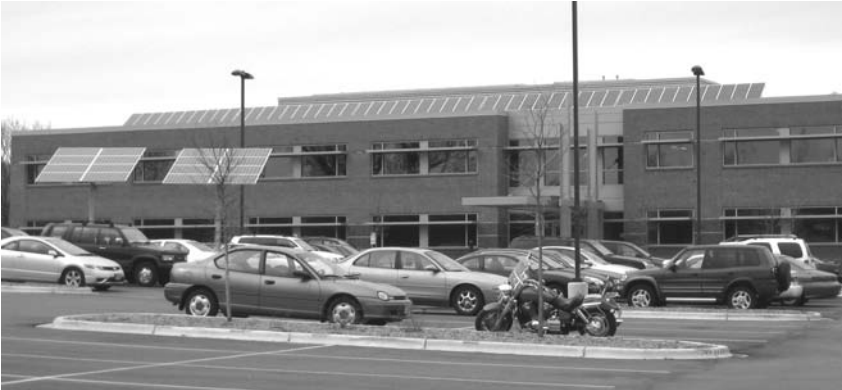
The Wisconsin Energy Conservation Corporation building in Madison, Wisconsin, is a LEED-registered project designed to achieve a LEED-NC Gold Certification. This building uses both solar electric and solar thermal technologies.
