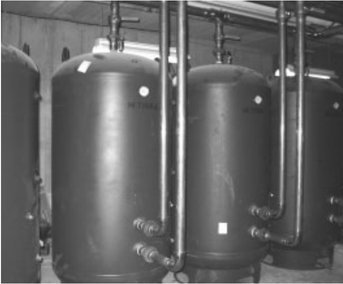
These photos show the Kalahari Resort & Convention Center, the pre-insulated piping that carries solar fluid from the solar panels to the Kalahari's hot water supply, and the 500-gallon pre-insulated storage tanks containing the solar heated water.
