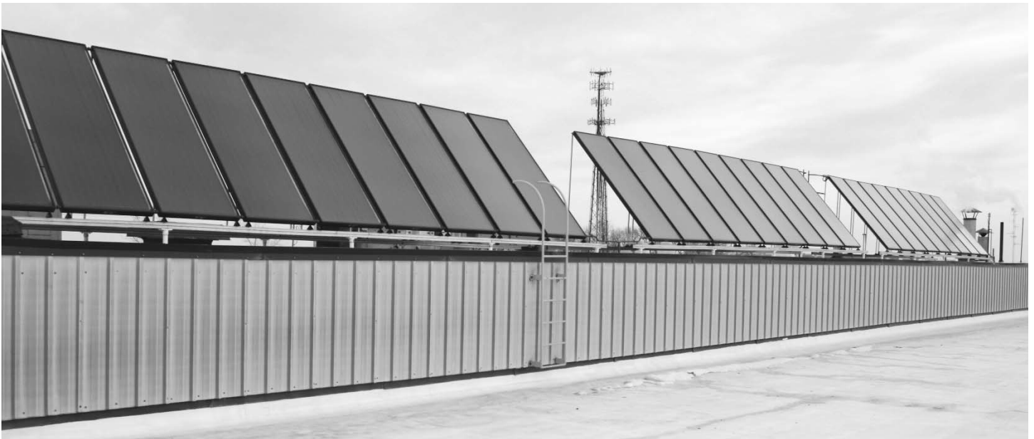
A maker of socks since 1904, Sheboygan-based Wigwam Mills now hosts a 27-panel system that preheats the water used in its color-dyeing process.
