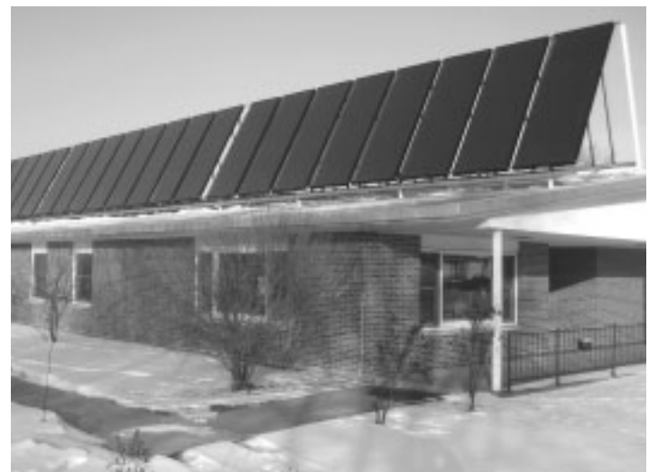
This 24-panel installation serves Baldwin Care Center, a nursing facility in Baldwin, WI. Installed by Area Mechanical, with assistance from Hot Water Products, this system will supply about 30 percent of the center's hot water needs.
