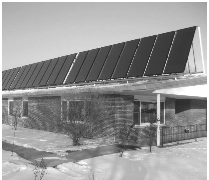
This 24-panel installation serves Baldwin Care Center, a nursing facility in Baldwin, WI. This system will supply about 30 percent of the center's hot water needs.
