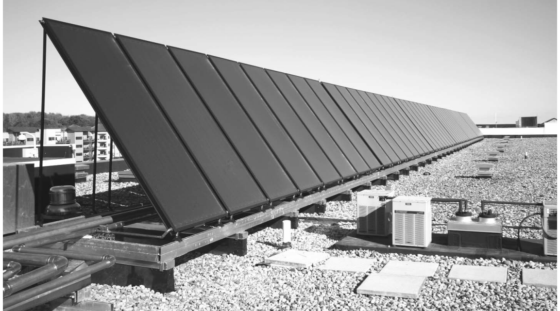
This 104-panel solar hot-water system atop the Kalahari Resort & Convention Center, Wisconsin Dells, is visible from Interstate 90-94. It provides over 3,000 gallons of hot water per day.
