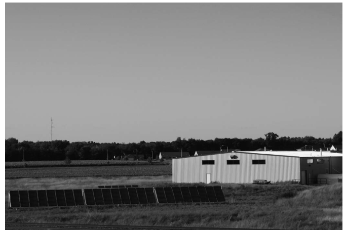
Central Waters Brewing Company in Amherst, Wisconsin installed a 24-panel solar hot-water system in March 2009.
