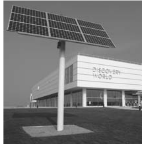
This 1.8 kW solar flag on a dual-axis tracker augments the educational mission of the Discovery World Museum in Milwaukee.
