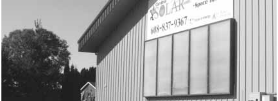
Glazed solar air collectors mounted on the south wall help heat the building for Advantage Plumbing in Cottage Grove.
