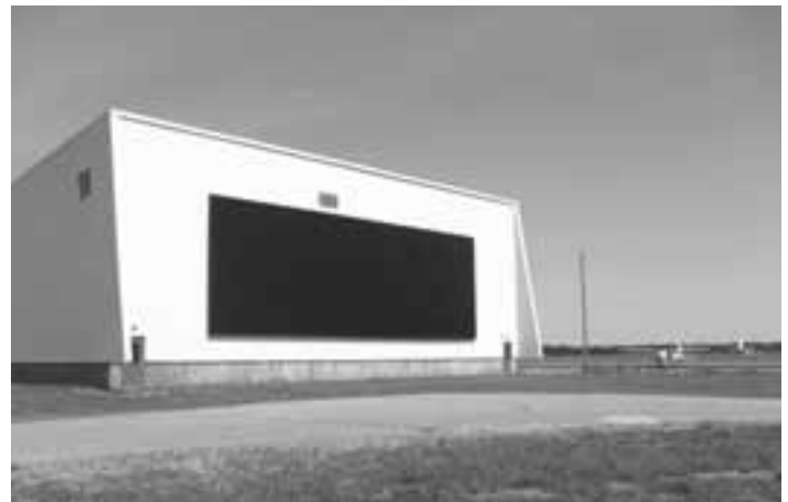
Unglazed, transpired air collectors installed on the south wall of a hangar at the Stevens Point Municipal Airport.
