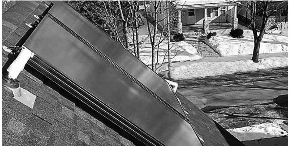
These roof-mounted flat plate solar collectors are connected by copper pipes to a heat exchanger plumbed to a solar storage tank, shown in the photo on reverse side.
