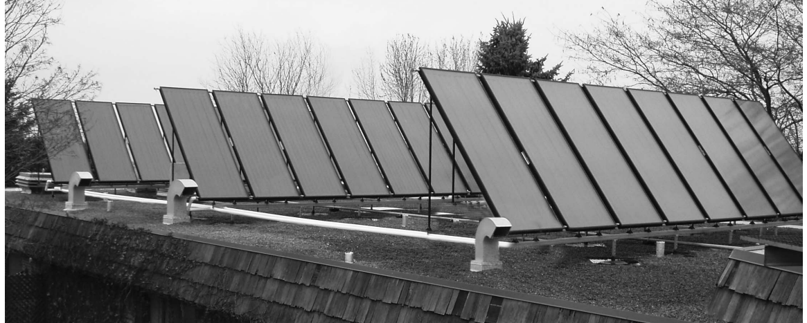
These solar thermal panels help control water heating costs for this Hammond, WI nursing home facility.
