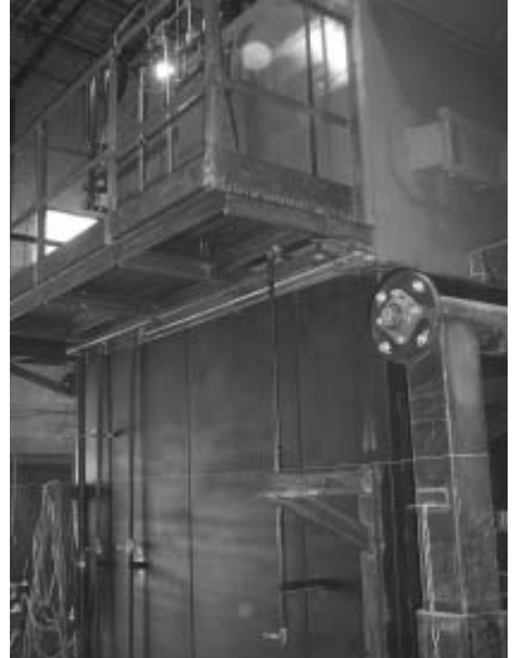
Superior Kilns' new wood waste boiler replaces two wood-burning boilers and two gas-fired boilers, increasing production and saving $185,000 per year in fuel costs.
