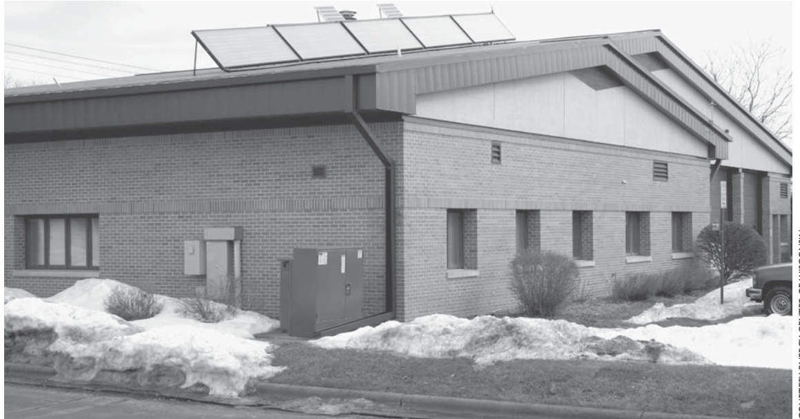
COURTESY ENERGY CENTER OF WISCONSIN
