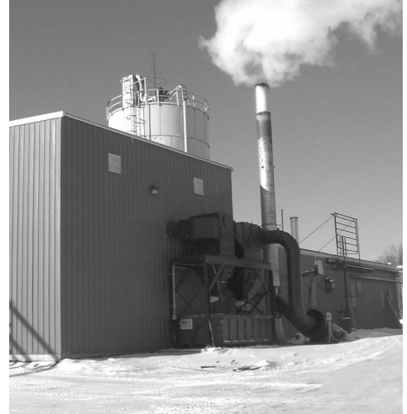
The new biomass energy system for Action Floors is up and running. This photo shows the biomass system building with its emission control equipment.
