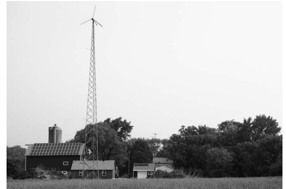
A combined solar electric and wind turbine system at TDL Electronics near Racine, Wisconsin. The 10-kilowatt wind turbine and the solar electric system powers TDL's office and facility.
