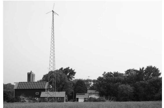
A combined solar electric and wind turbine system at TDL Electronics near Racine, Wisconsin. The 10-kilowatt wind turbine and the solar electric system powers TDL's office and facility.
