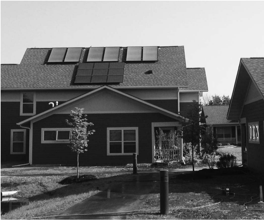
Many residents chose to incorporate solar energy during the building process. Shown here are six solar hot water heating panels and a square grouping of nine solar electric (PV) panels.
