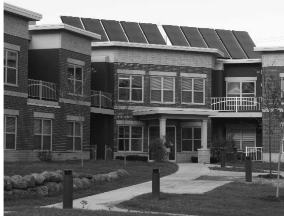
Ten solar panels sit atop the Yahara River View Apartment building. A solar hot water system like this can provide 50 percent to 75 percent of a building's domestic hot water needs.
