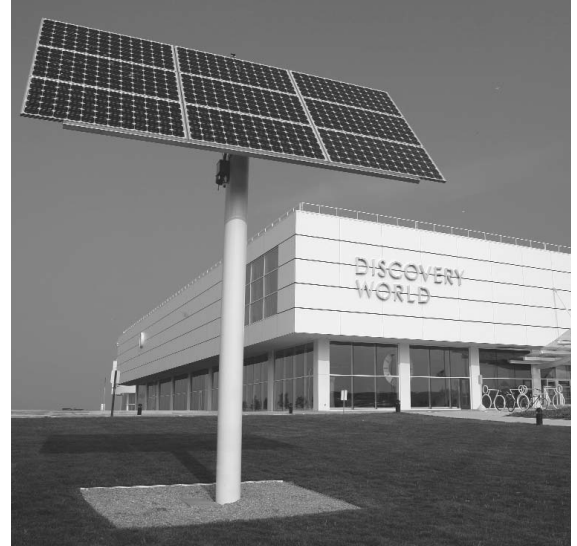
This 1.8 kW solar flag on a dual-axis tracker augments the educational mission of the Discovery World Museum in Milwaukee.
