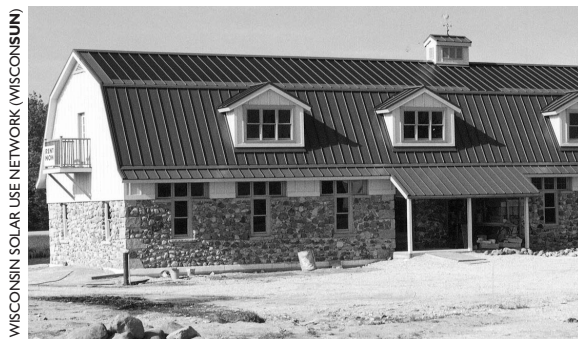
(right) The Ritger Law Office in Random Lake, Wisconsin, is connected to the grid but stores solar electricity from its solar electric roofing panels to provide uninterrupted power for computers, telephones and lighting.
