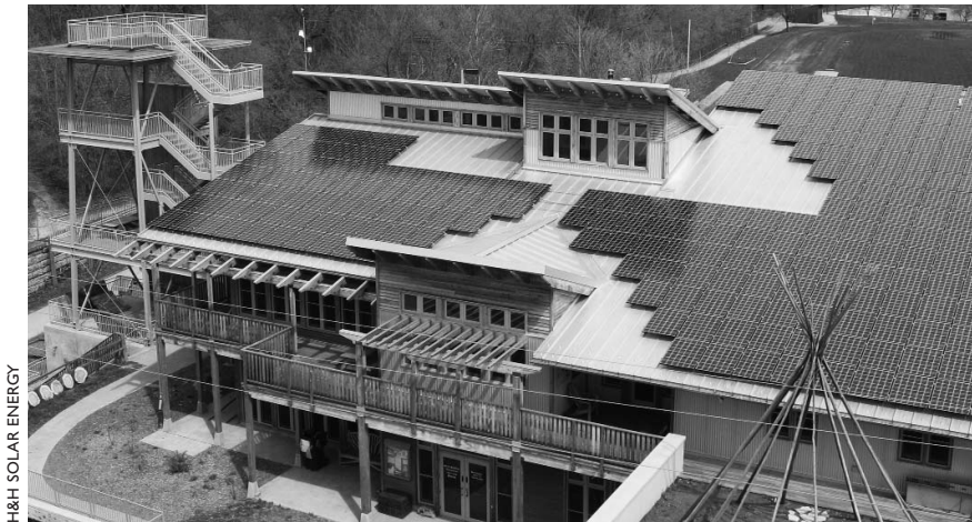
(top) The Urban Ecology Center in Milwaukee, Wisconsin features a fixed-mounted 44.4 kW system on its roof.
